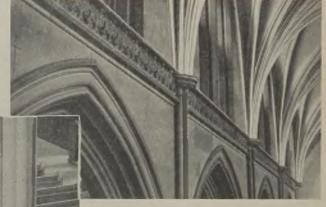
Above: Heating pipes, almost unnoticeable, have been run round the tops of the pillars to overcome the natural chimney effect. Left: Special low radiators at the base of the pillars for warming the centre of the building
