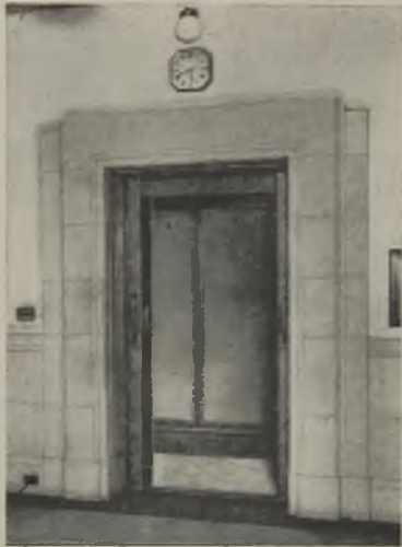
One of eight Lifts installed in Bolton Town Hall
