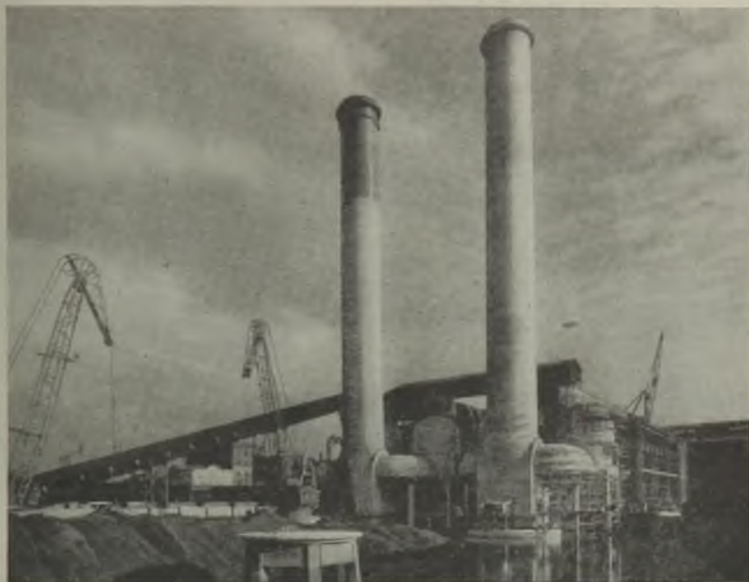
REINFORCED CONCRETE CHIMNEYS
