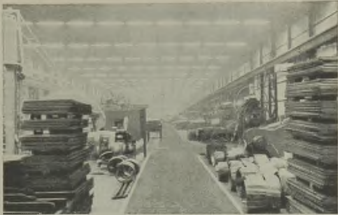
Fluorescent lighting in a blacked-out rolling mill
