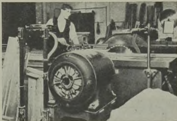
Crompton Parkinson "Klosd" motor driving wood-working machinery in a converted sawmill
