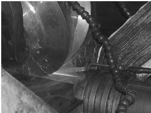
Fig. 6. Pressure welding operation
