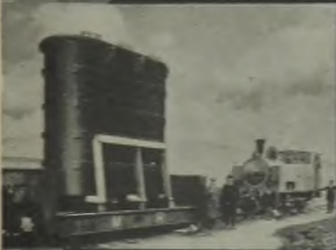
The first 18,500 kVA, 3-phase 22 kV Transformer made in this Country.
