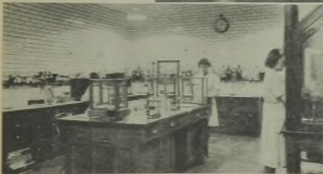
Above: The load on the E.R.A. impact machine (left-hand of picture) can be varied from 1/2 ft.-lb. up to 13 ft.-lb.; mechanical testing includes torque tests (right-hand) and blow and transverse testing for telephone cradles and handles. Left: A feature of the chemical laboratory is the absence of bench sinks, water being available at any point, and waste removed by continuous water channels
