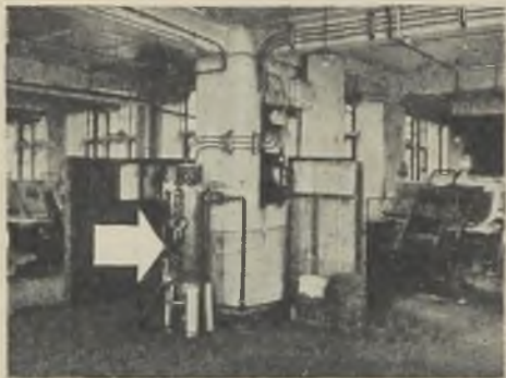
B & A Steam Boiler 150kw, supplying steam to Knitwear Presses
