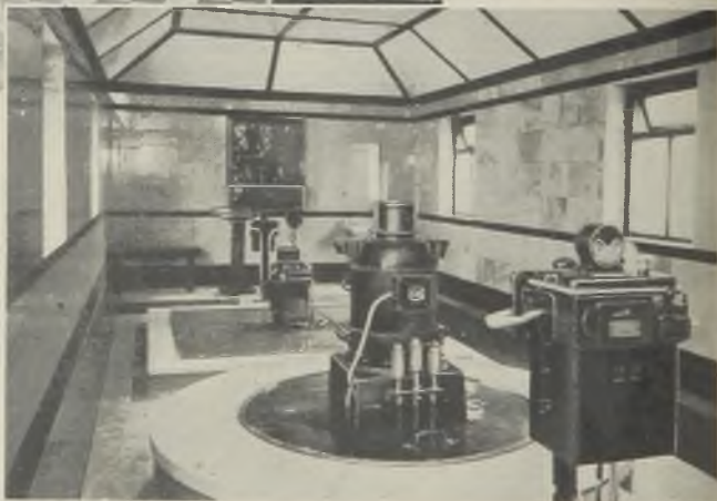
Above: The 220-HP high-speed prime mover is directly coupled to a 175-kW 400-V 3-phase alternator and exciter, and main distribution is via an open-type switchboard equipped for automatic voltage regulation
