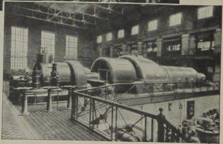
$1,250 kW 1,500 r.p.m. "Metrovick" 2-cylinder Turbo-Alternator Set.
