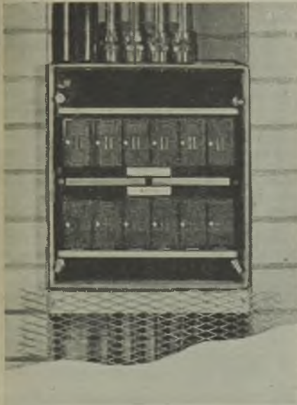
Accommodation of rising main system in chase
