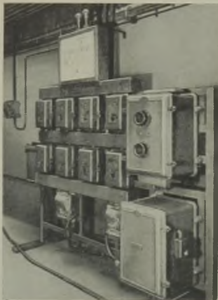
Factory sub-distribution board for pulverising plant showing fuel circuit diagram
