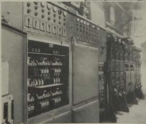
Convertor blower house distribution board showing one of the blowers and (left) sequence control board No. 2 and foundry No. 2 distribution board
