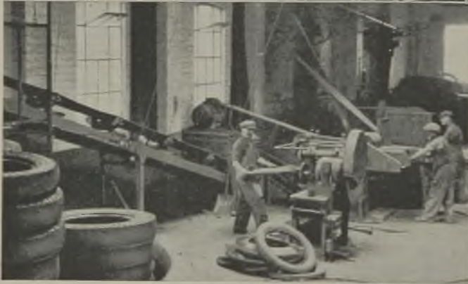
Equipment for the initial preparation of the material, i.e. de-beading and chopping machines, is installed in an annexe to the main plant room
