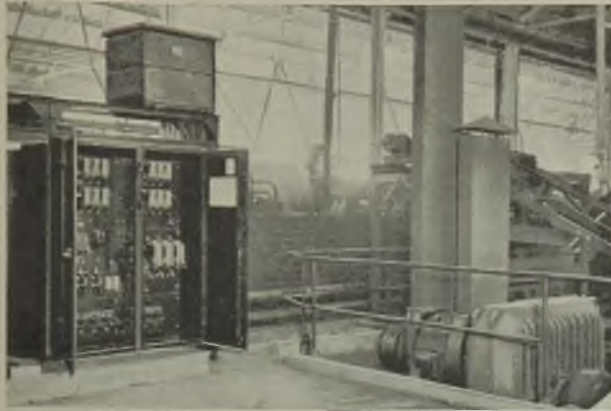
Above: Each cracking mill is driven by a 150-HP pipe-ventilated motor; all the starting equipment for this motor is housed in an iron-clad cabinet with hinged doors Right: A motor-driven travelling hopper (above) discharges the mixture into steam-heated revolving spherical digestors below
