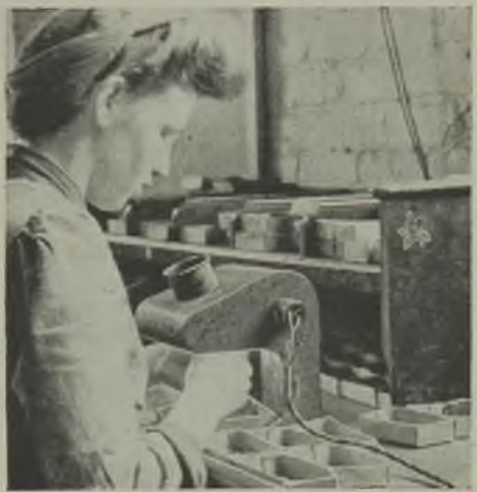
Inspecting tungsten contacts
