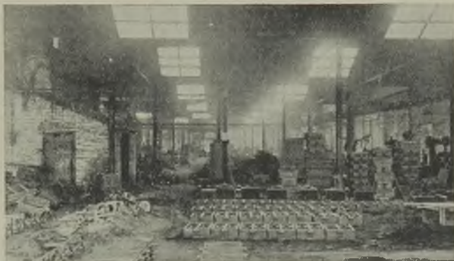
A foundry lighted by "Mazda" fluorescent lamps
