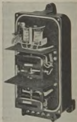
Fig. 1.—Standard type of "Rythmatic" control switch
