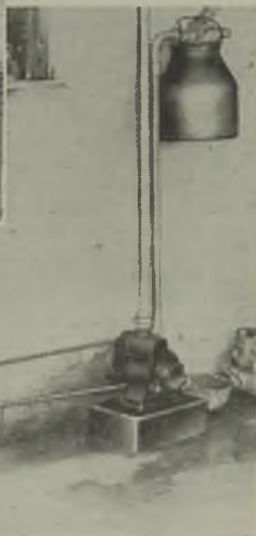
Milking equipment : Above, sterilising boiler and chest. Left, two-unit milking machine. Below, motor - driven vacuum pump
