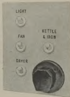
Fig. 2.—Sub-circuit control unit
