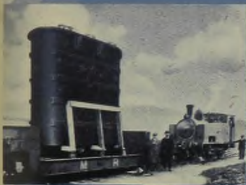
The Great 18,500 kVA Transformer — 66 kV, manufactured in this Country.
