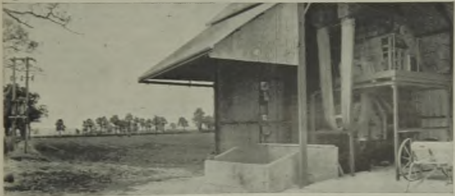
The modern grain dryer is one of the finest examples of electric service to agriculture ; supply point on left
