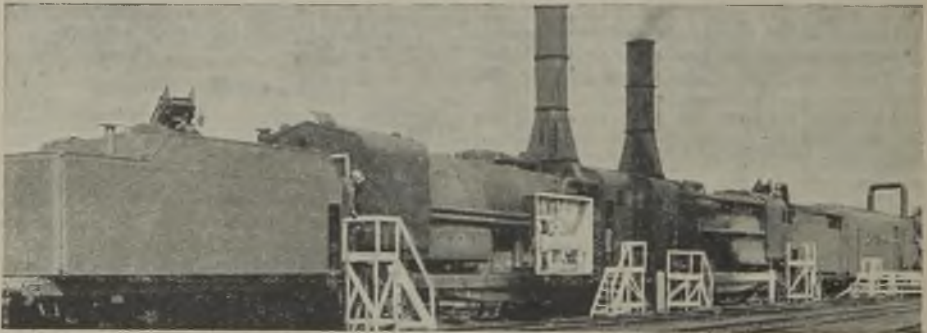
Generating and power sections of a 3,000-kW ten-car train power unit
