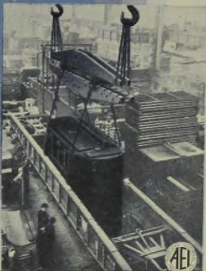
75 MVA, 3-phase 66 kV Transformer recently supplied.
