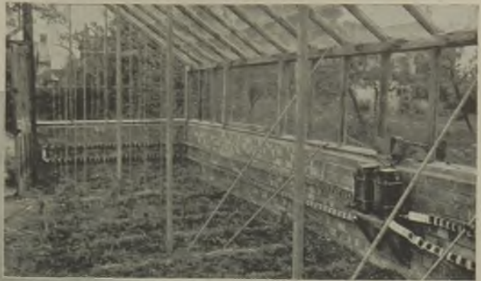
Bare elements are operated at low-voltage in this greenhouse heating scheme, so that it is permissible to use water freely
