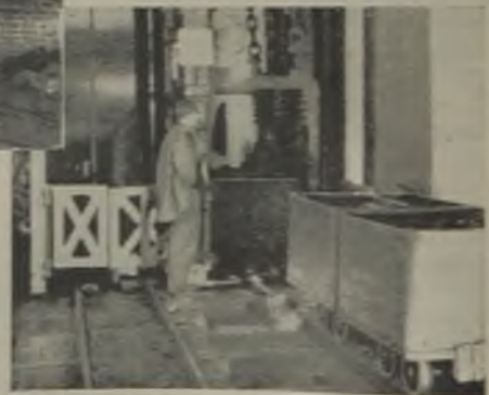
Now the whole of the mine product is worked from one shaft (downcast): pit top (left) and pit bottom (right) of downcast shaft
