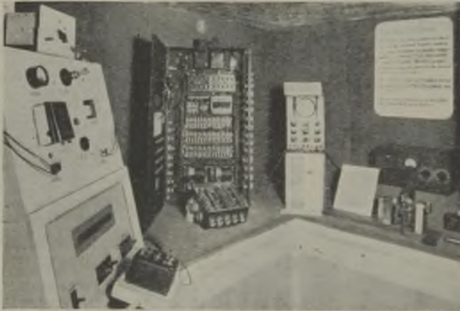
Automatic telephone unit for testing complicated wiring systems
