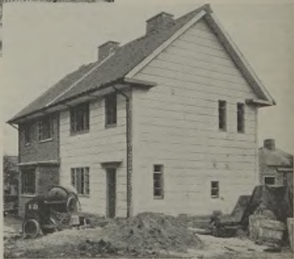
The steel framework and (right) the houses nearing completion, showing brick and asbestos coverings
