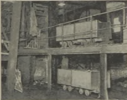
Now the whole of the mine product is worked from one shaft (downcast): pit top (left) and pit bottom (right) of downcast shaft
