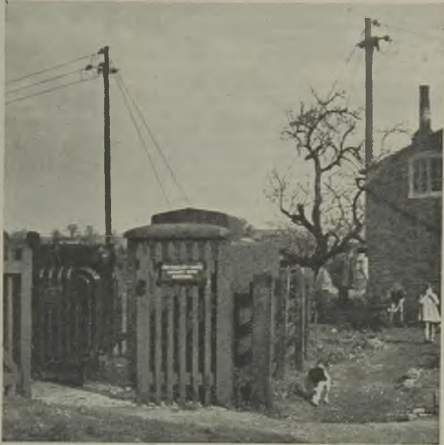
Typical rural substation, with 100 kVA transformer, at Campton
