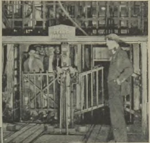
The upcast shaft is used for men and materials other than coal: pit top (above) and pit bottom (left) of upcast shaft
