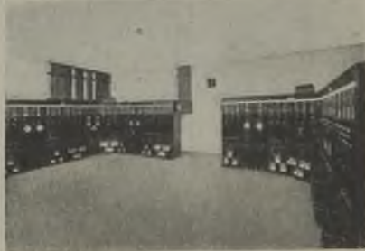
Remote Control Board for Sections 2 and 3 Switchboards Illustrated above
