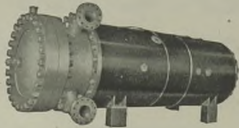
HIGH PRESSURE FEED WATER HEATERS HT 2016 2
