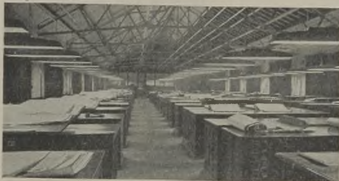
Fluorescent lighting at an L.M.S. Railway drawing office
