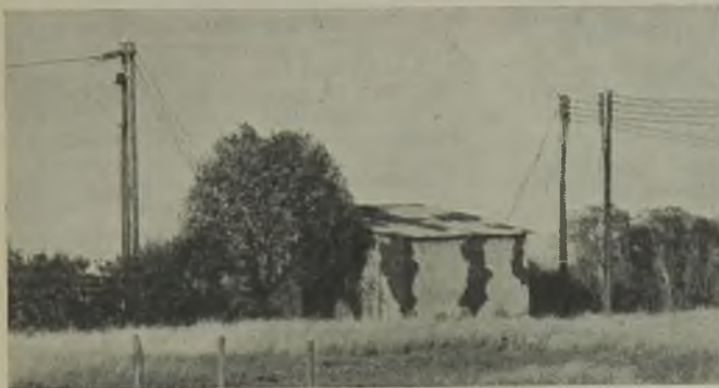
At several points in each area a h.v. supply terminates at a switch in a transformer house from which the l.v. lines radiate to the wells. Right: An impression of orderliness is given despite overhead lines, roads and wells
