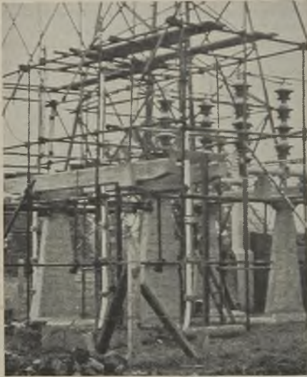
Above : The cables rise out of the ground and up the concrete pedestals of the special switching structure where the cable ends are bottled off.
