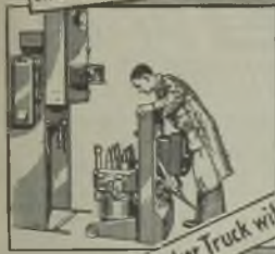
Circuit Breaker being racked down for isolation
