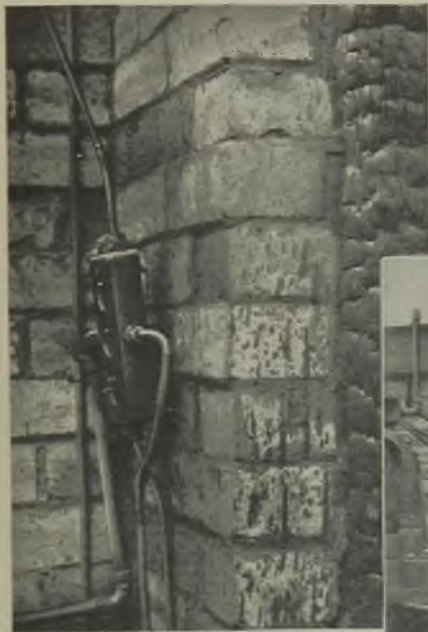
Above: "Pyrotanax" cable and conduits entering a switch-unit in burnt-out warehouse. V.i.r. cable inside the conduit is completely destroyed due to the fierce heat, which is indicated by the charred timber door post.
