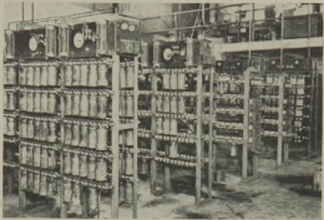
The colliery has a well-appointed charging room for the miners' electric lamps
