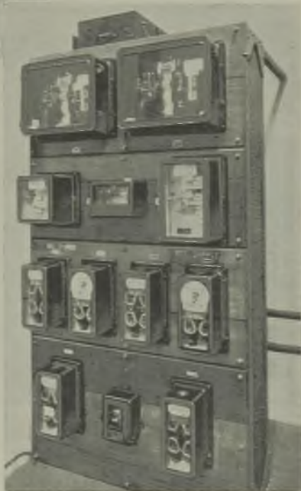
In addition to normal metering the two supplies for the substation are summated, and in one of the substations the two substation supplies are also summated by the top meters
