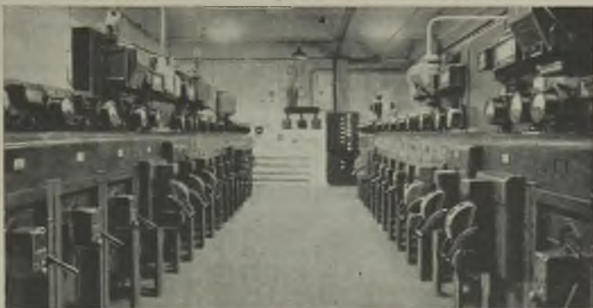
In some cases the l.v. switchgear is imposingly set out in two facing lines
