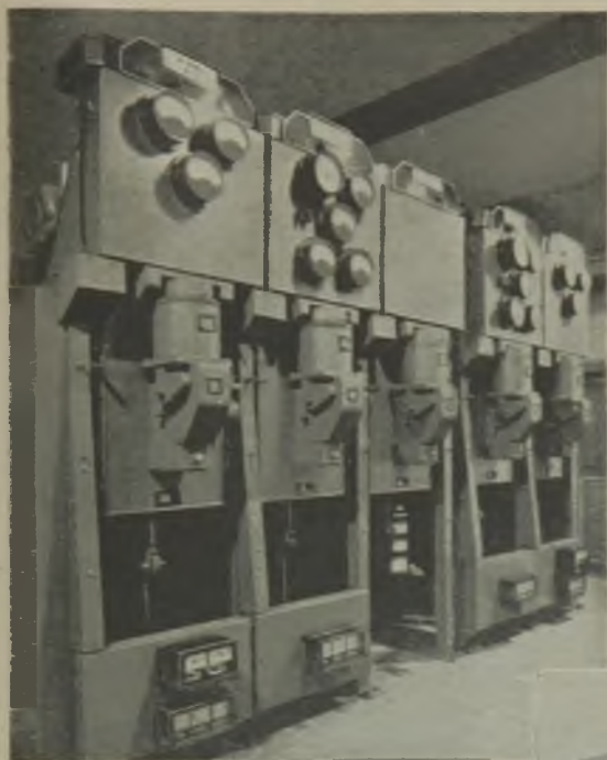
The main factory substation switchgear is of the spring-closing vertical-isolation type
