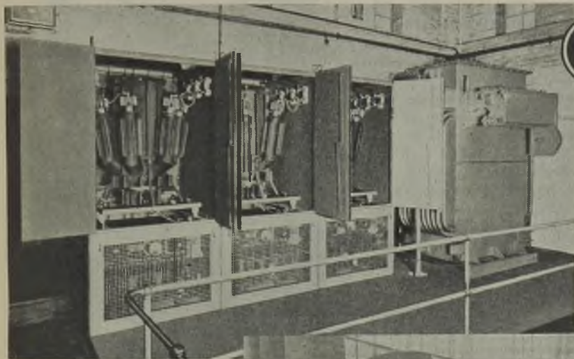
Three Steel-bulb Rectifiers operating in parallel off one transformer, for power supply to a dockyard.
