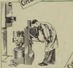
Circuit Breaker Truck withdrawn from cubicle
