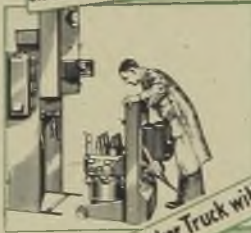
Circuit Breaker being racked down for isolation
