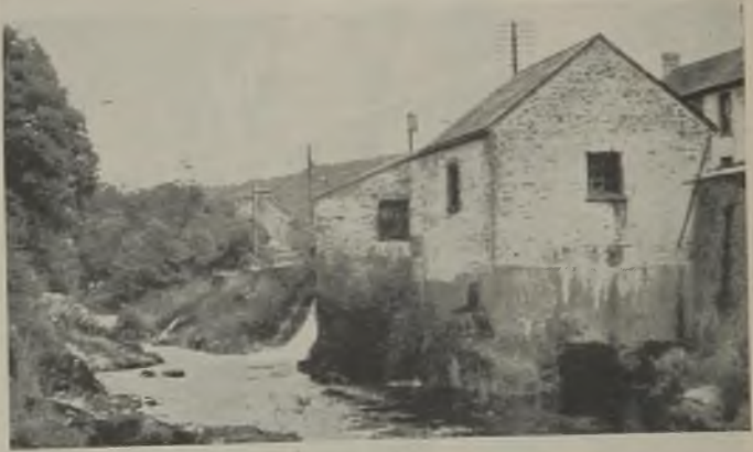
Llandyssul hydro-electric station
