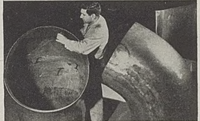
Hand-finishing copper vent stack elbows
