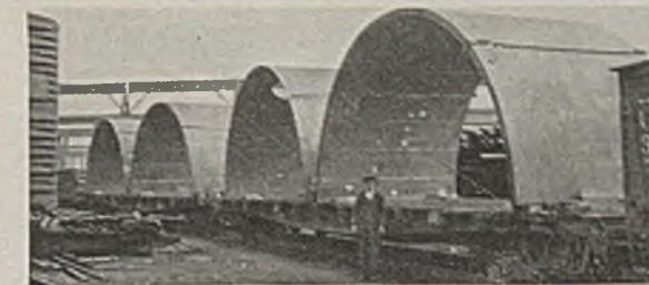
Shell plates for top section of tower were shipped in parts as shown above, for field erection.
