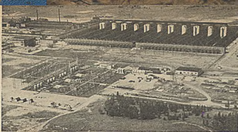
Mead aluminum reduction plant of the Permanente Metals Corp. at Spokane, Wash., where the first Kaiser aluminum was produced last month. Annual capacity is 216 million pounds of aluminum ingot
