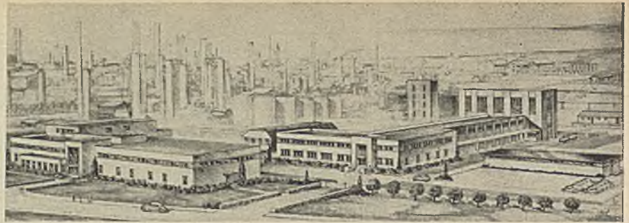
Proposed developments at California Research Corp., Richmond, now getting under way. Drawing shows additions to the present laboratory and office buildings (left) and the new process laboratory and pilot plant building (right)
