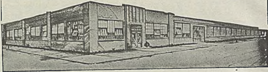
MODERN PLANT DOING MODERN REBUILDING
