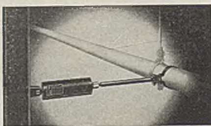
Single-spring preloaded sway brace
