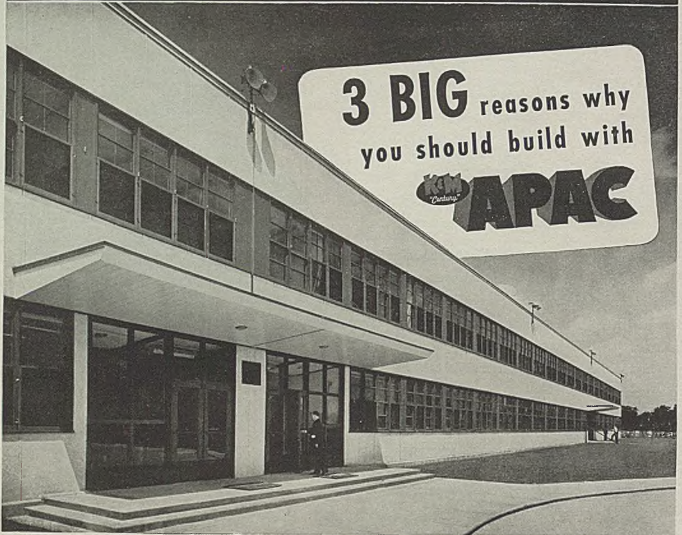
● APAC, used as exterior siding on this huge administration building, combines up-to-the-minute design with maximum durability. Design and Construction by The Austin Company.
