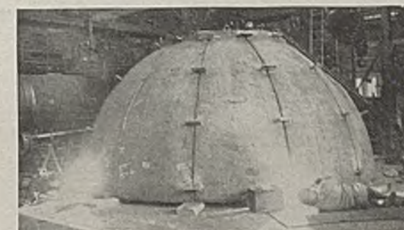
Segments of the hemispherical head were drawn together and shop-welded into two sections at the B&W plant.
