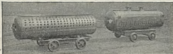
Sludge Heater for Sewage Treatment
