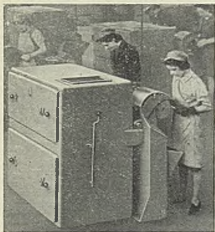
Polishing machine with standard "Drymat" equipment in a large aero-engine works. The hand-shaker, for depositing the lighter dust, is seen on the front of the unit.
