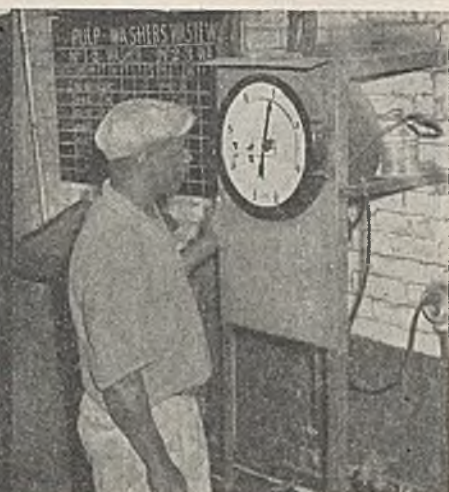
MODEL R MICROMAX FOR pH OF HOT WASH LIQUOR AFTER CHAR FILTERING, NATIONAL SUGAR REFINING COMPANY
