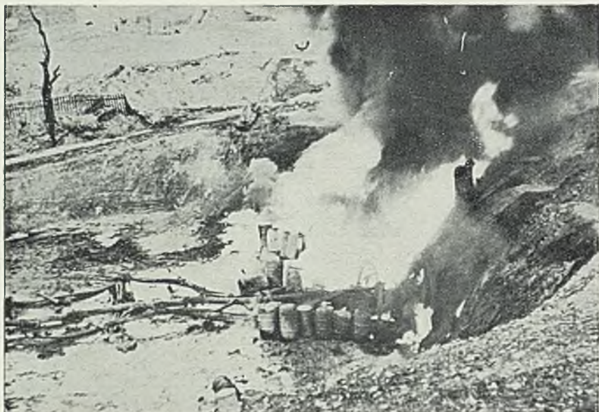
FALMOUTH. STEPS TAKEN TO CONFINE THE CATARACT FIRE BY FORMING A DAM OF OLD OIL DRUMS, EARTH, ETC.
