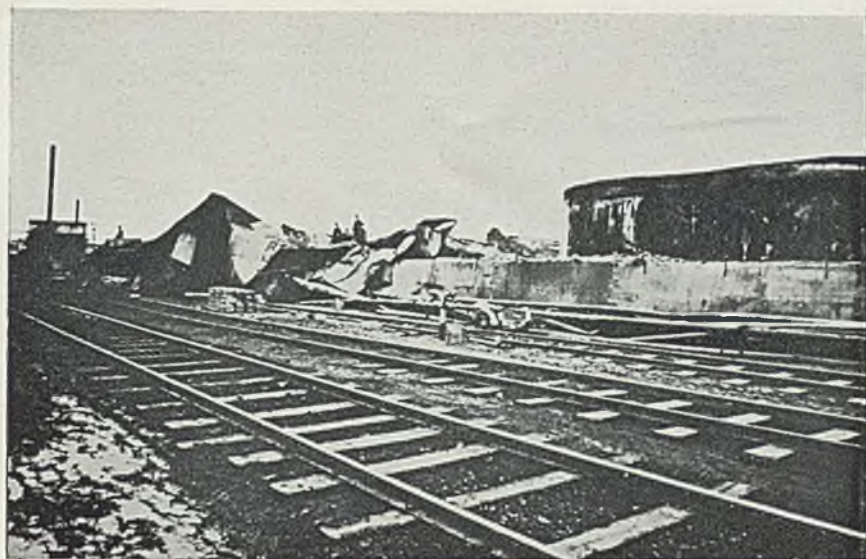
AVONMOUTH. VIEW OF TANK WHICH HAS COMPLETELY COLLAPSED.
