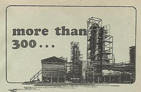
100,000 pounds of ethylene per day is the capacity of this plant, designed and built by Lummus.
