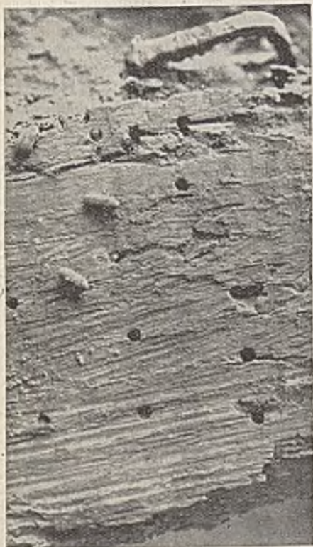
Fig. 3. Death-watch beetles on the surface of an infected oak beam (approx. nat. size).
