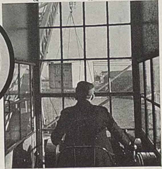
Interior view of crane-cab at eastern railroad pier, showing compact EC&M Master Switches conveniently grouped within easy reach of the operator.
