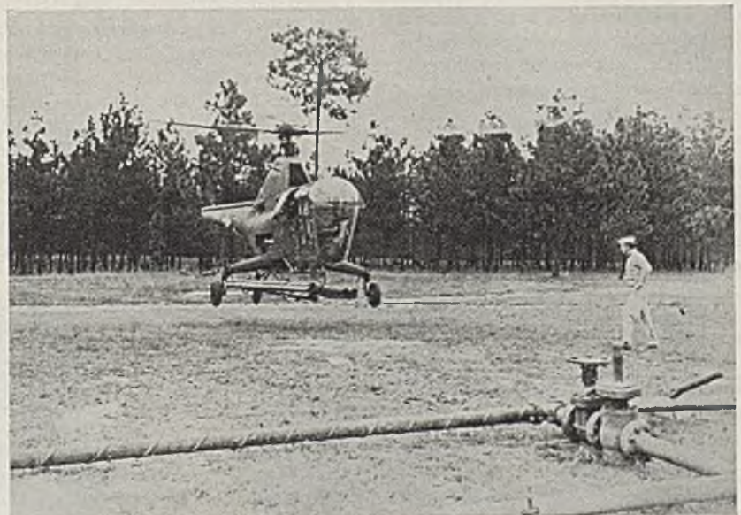
HELICOPTER AIDS PIPELINE CREWS: Army petroleum distribution experts used helicopters in building pipelines through impassable swamps during secret war-time tests. Photo shows how the helicopter delivered 20-foot sections of pipe to construction crews in Louisiana swampland. The craft also carried other equipment to the crews. NEA photo
