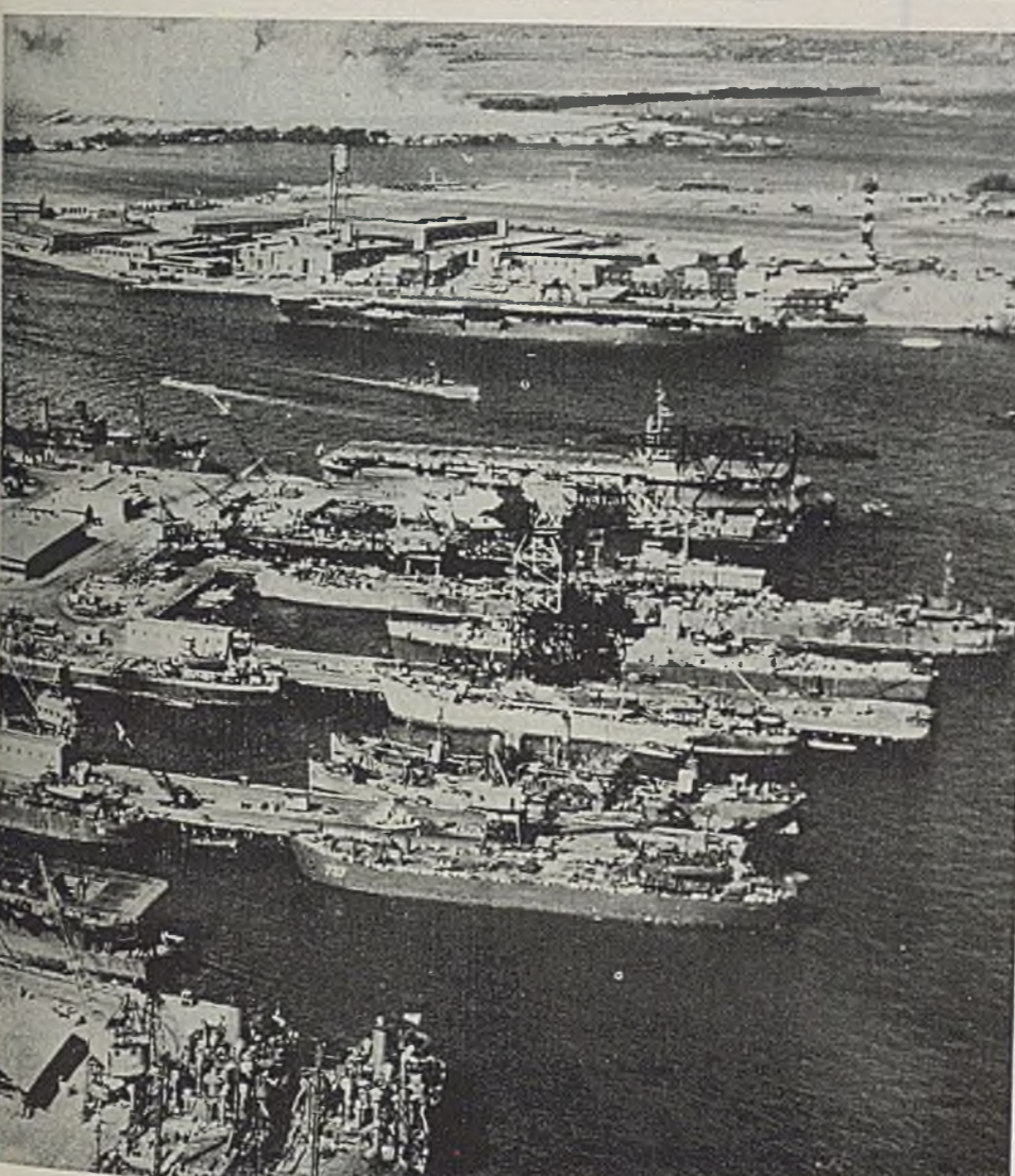
Visible evidence of United States sea power is seen in this aerial view of Pearl Harbor, the Navy's powerhouse of the Pacific. Shown are three aircraft carriers, half a dozen LST's and numerous other craft as well as some of the construction carried out during the war. U. S. Navy photo from NEA
