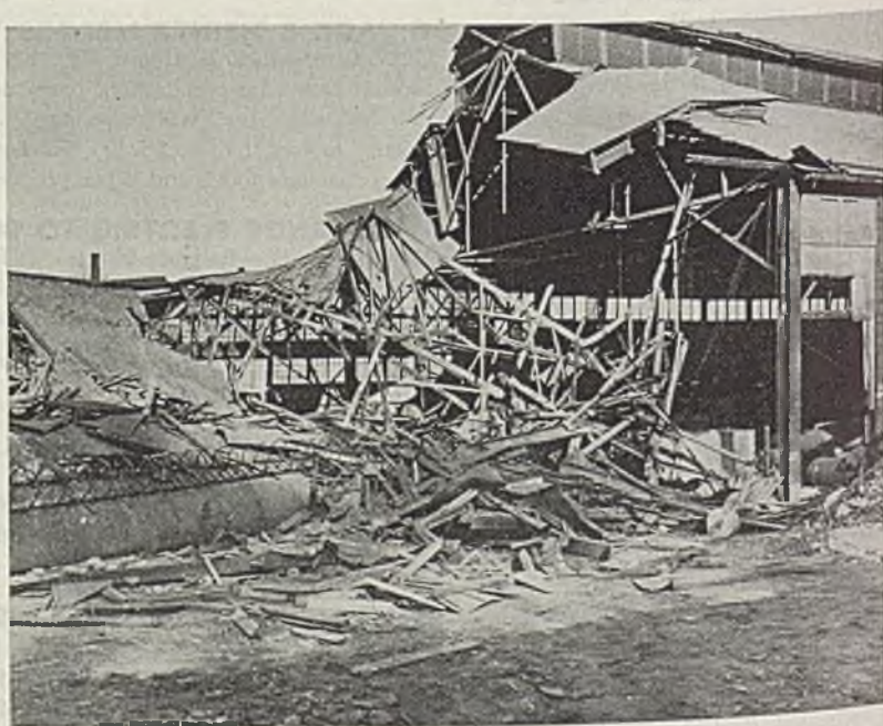
ACCIDENTAL DEMOLITION: Thousands of dollars worth of machinery was damaged when a 300-foot high brick-lined steel smoke stack fell the wrong way during wrecking operations of the old Pencoyd Iron Works outside of Philadelphia. The plant, operated during the war for export tonnage, is being torn down, but the building shown above was being used for storage purposes. NEA photo
