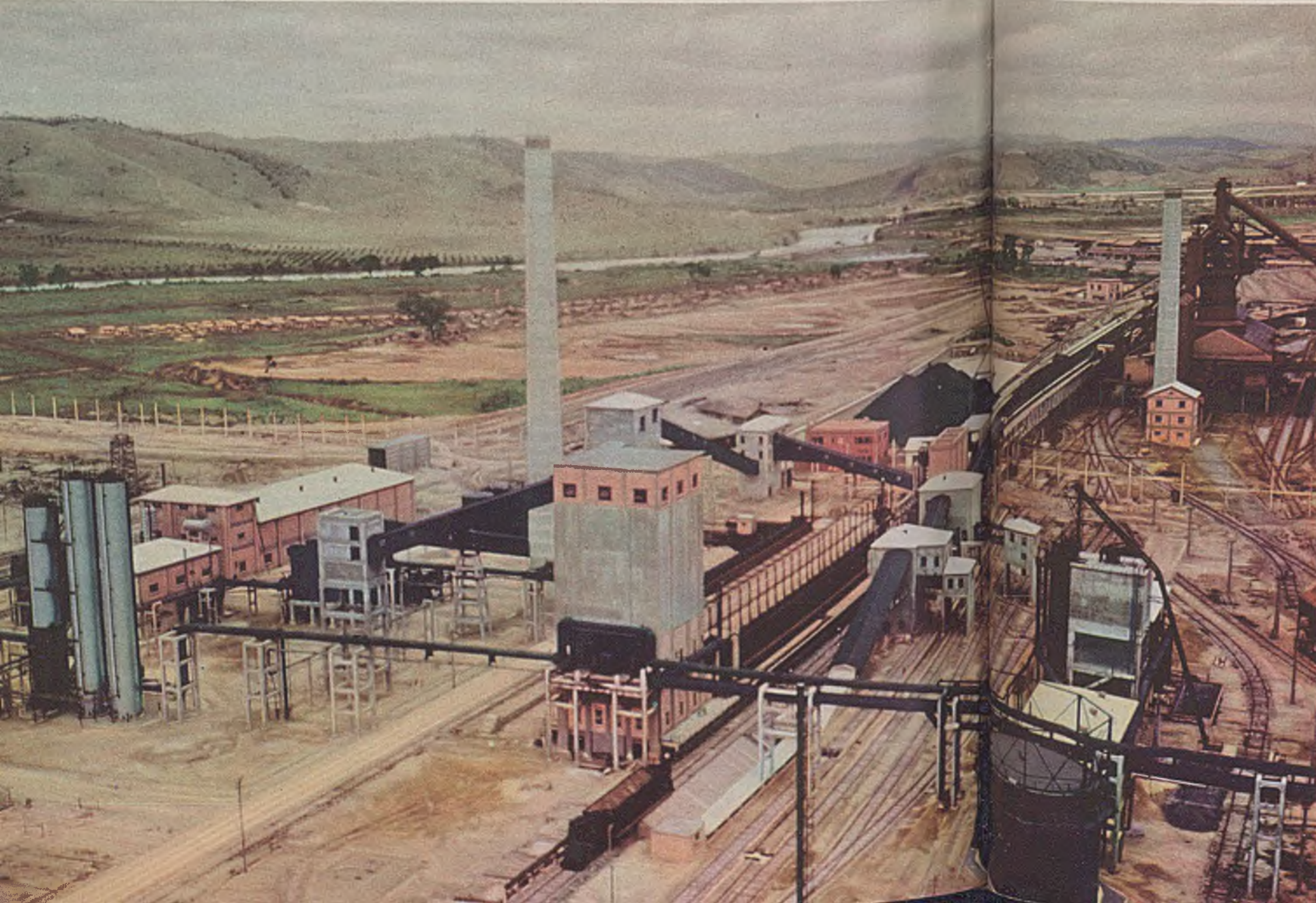
Koppers-Becker Underjet Coke-Ovens with Waste-Gas Recirculation and Koppers Byproduct Plant at Volta Redonda, Brazil.
