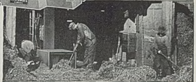
Low level installation of American Crusher
