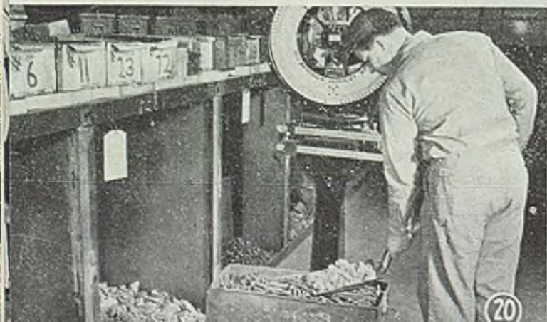
Fig. 20—Meanwhile, raw materials for the alloy to be cast (in this case, Type 347 stainless) are being accurately weighed out, melted down in Ajax induction furnaces and cast into small “stick” pigs
