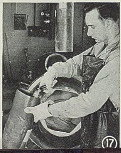
Fig. 17—The flask containing the wax assembly then is carried to the next department on an overhead hanger-conveyor where it is filled with a chemically-hardening investment material. This material, comprising tetraethyl silicate, crushed firebrick, silica sand and alcohol, is mixed on the floor above. The small mixer shown at the operator's right is filled as required by means of a chute
