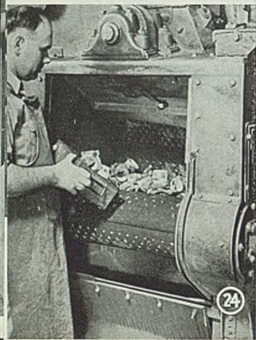
Fig. 24—Castings then are shot-blasted to remove scale and remaining investment material. This step would be eliminated in the case of castings with thin edges. Castings then are subjected to rough inspection to remove those with obvious defects
