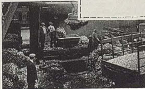
Typical scrap yard installation of American Metal Turnings Crusher where long curly turnings are reduced to short shoveling chips.
