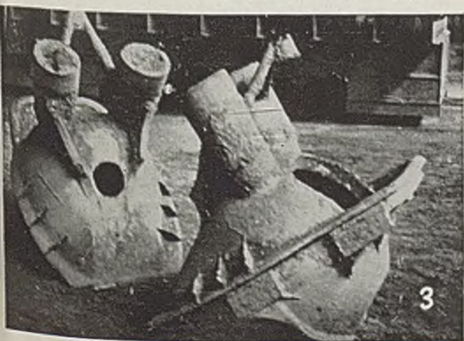
Fig. 1—Cope view of tank track castings
