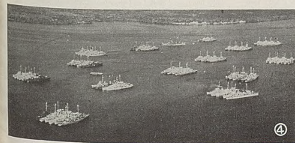
Fig. 4—More than 100 destroyer escort vessels shown here in St. Johns River at Green Cove Springs, Fla., are being preserved against corrosion for many years to come. A crew is kept aboard one of the six ships in each group to service preservation equipment
