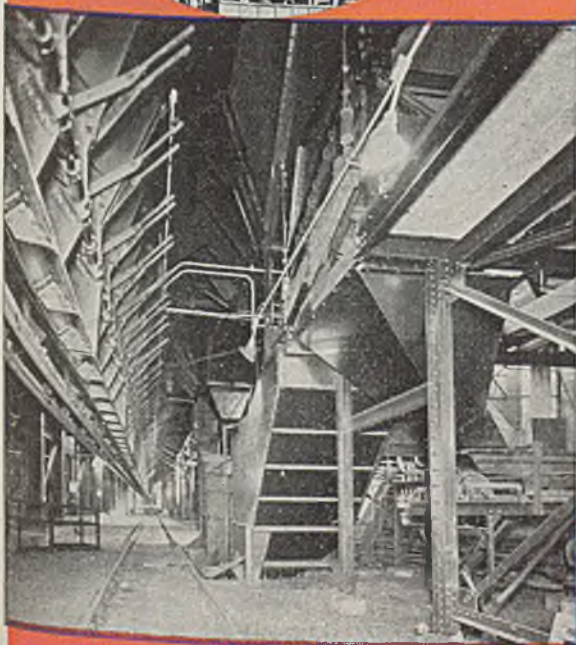
Stockhouse, showing McKee hand-operated gates.
