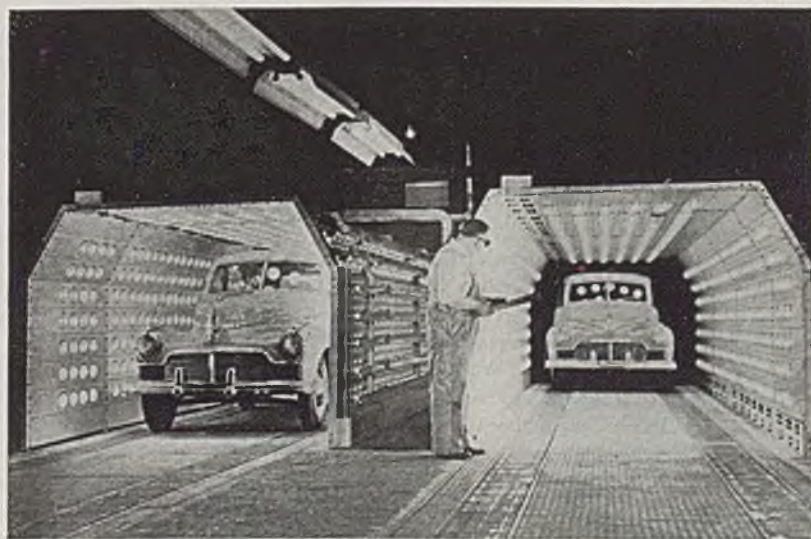
SPEEDS PAINT DRYING: An assembly line installation of infra-red ovens that reduces the time of paint touchup processes by two-thirds has just been revealed by Studebaker Corp., South Bend, Ind. The 32-foot ovens, each containing 800 lamps on 20 different parallel circuits, are operated to dry primer coats of paint. Enamel is then applied and the surface baked in a conventional steam tunnel oven
