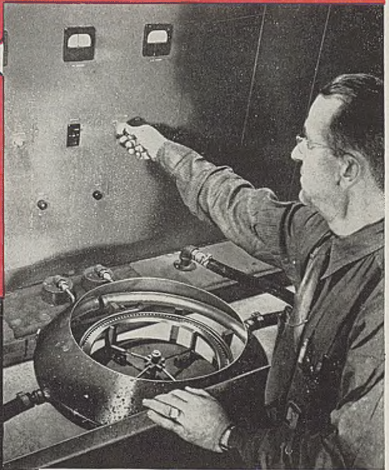
▲ G-E 50 kw electronic heater, used at Studebaker's South Bend plant
