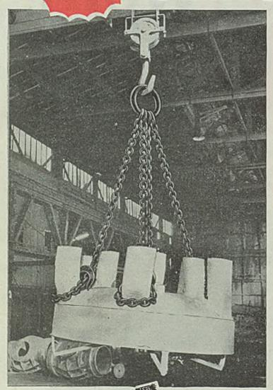
FOR dangerous overhead lifting, particularly where shock loads must be handled, safety recommendations call for wrought iron sling chains. Cleveland Sterling Grade Wrought Iron Sling Chains provide the highest degree of protection against sudden breakage. Made only by highly skilled chain makers, Cleveland Sterling Grade Sling Chains are unsurpassed for heavy-duty lifting where the safety factor is paramount.
