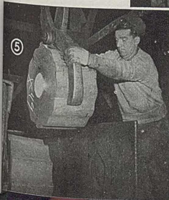
Fig. 4—Following "nicking" operation, ingot is brought to this "breaking" press where sliced blocks are pried off
