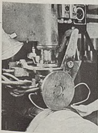
Fig. 2—Welding cross-over tubes to flame tubes by atomic-hydrogen process. Photos in both Fig. 1 and 2 were taken at ITE Circuit Breaker Co., sub-contractor fabricator
