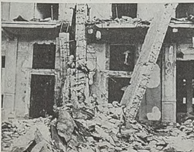
VAULTS SURVIVE ATOMIC BOMB: Bank vaults in Hiroshima survived the blast and heat of the atomic bomb despite the fact the reinforced concrete bank building was blasted to rubble. Shown at left is the
