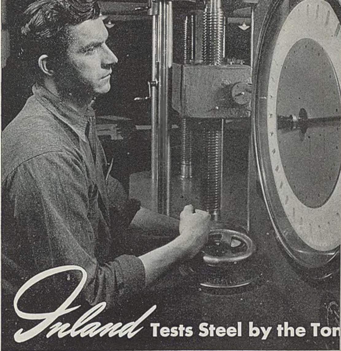
Operator determining physical properties on one of the many tensile testing machines in the Inland laboratory.
