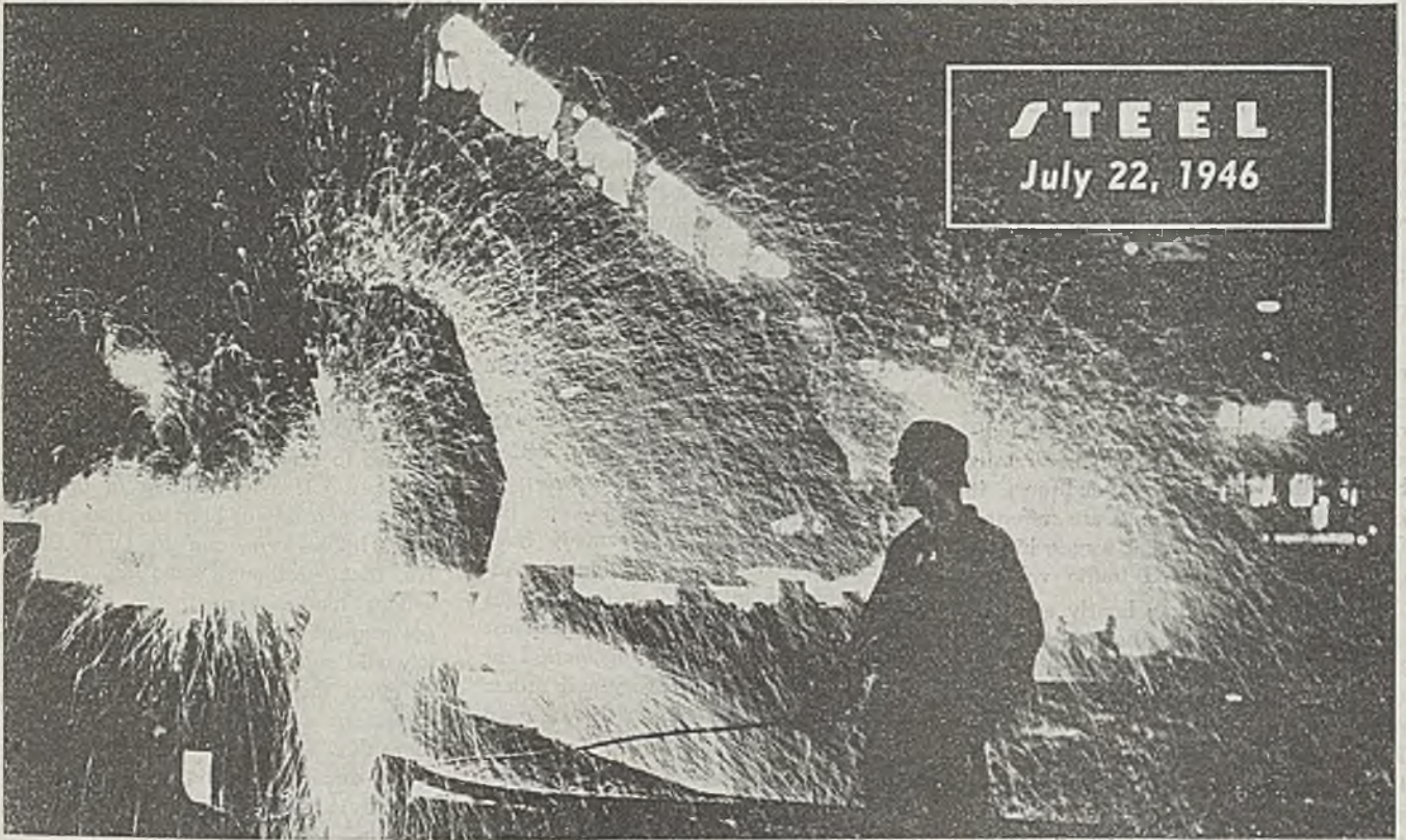
Newly-rolled steel rails go under giant saws to be cut to proper length for track replacements at the Edgar Thomson Works of Carnegie-Illinois Steel Corp. at Braddock, Pa. Workmen at Edgar Thomson see the display of pyrotechnics every few minutes as rail production is pushed to meet the unprecedented demand
