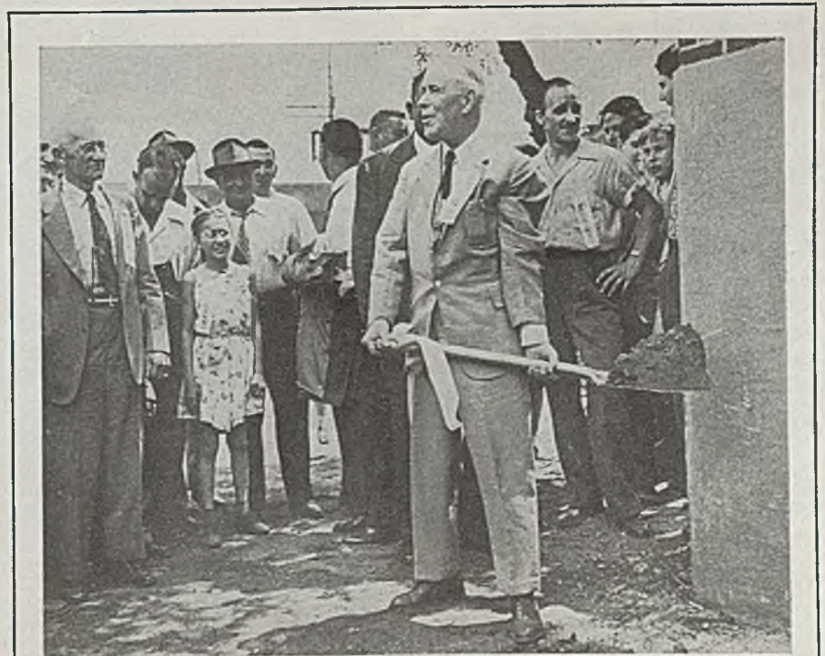
STARTS NEW PLANT: As Robins Conveyors Inc. celebrated its 50th anniversary by announcing construction of a new manufacturing building at the Passaic, N. J., plant, Thomas Robins, founder of the company, turns the first spade of earth
