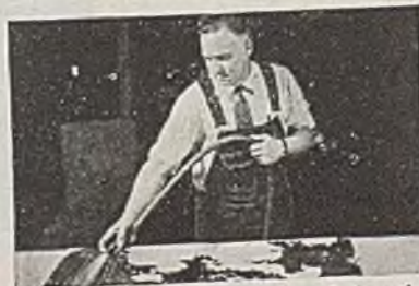
3. Rinse with weak ammonia solution—the reproduction, in white line for easy seeing, is on the material.
