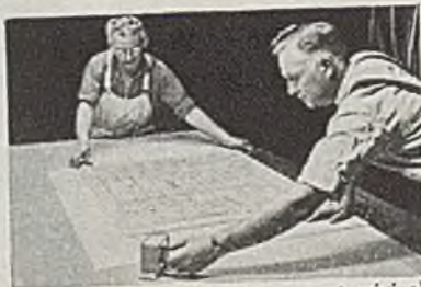
2. Place translucent or transparent original in contact with Transfax coated surface and expose to bright light.
