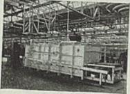
An II continuous tube type special atmosphera furnace.
