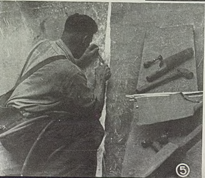
Fig. 5—Welding conical-shaped bottom of a lead-lined Foamite tank. Tools needed for work are shown alongside worker. These consist of a shave hook, wooden dressers for dressing down lead, hammers, and lead welding rods. Also included is a flapper of sheet lead for smoothing out lead lining
