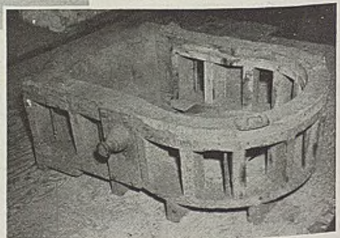
Fig. 1 (above)—Steel, all-welded follow board of more serviceable design, weighs only one-third as much as former unit
