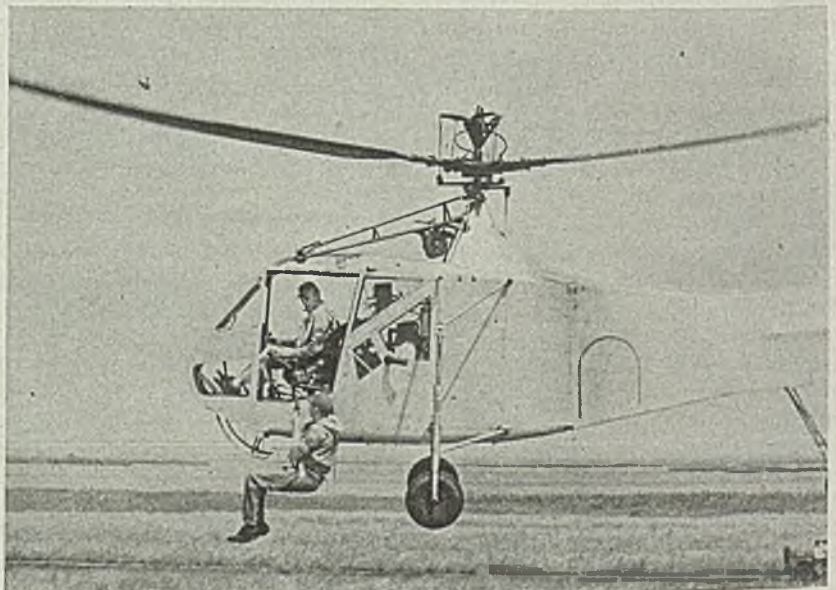
NAVY TESTS HELICOPTERS: Helicopter Development Squadron Three of the Navy is putting "windmills" through their paces at Floyd Bennett Field, N. Y., in an attempt to find their greatest value to the Navy. Apparent uses now are air-sea rescue, gunfire observation, antisubmarine patrol and liaison work. This photo shows a "sea rescue" being demonstrated on land; a line from a power hoist on the helicopter is dropped to the "victim," who fastens the line to his life jacket and is pulled aboard the aircraft. NEA photo
