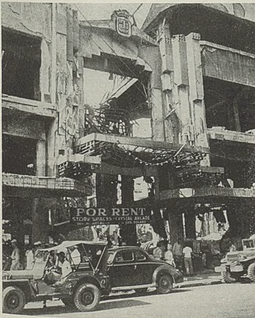
Manila, once proud "Pearl of the Orient," is only beginning to emerge from the ruin and destruction visited upon it during the war. Now temporary buildings are being constructed as the city strives to get back to normal. Above office building on the Escolta is typical of the destruction caused by bombings. NEA photo
